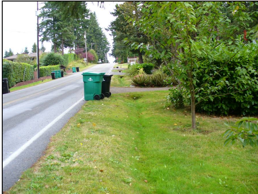
Photo 2, facing eastward along NW 180 th Street, showing the swale-like, non-stream streetside storm drainage system which discharges to Bear Reserve (Oct. 2, 2008).
